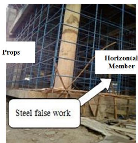
Figure 98. Steel Props.
