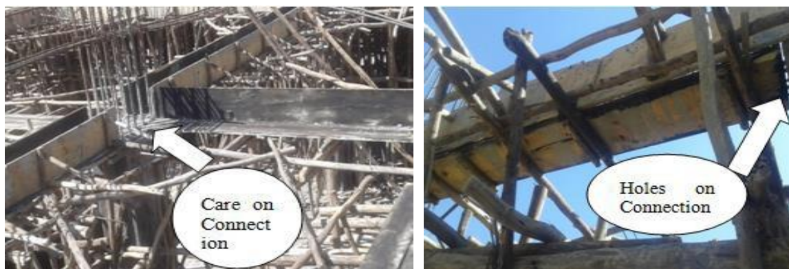
Figure 7. Beam Formwork.
