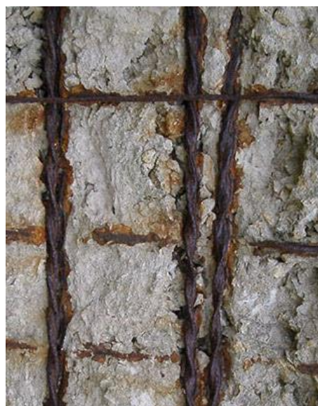
Figure 7. Cracks Due to Corrosion.
