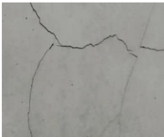
Figure 1. Hairline Crack.
