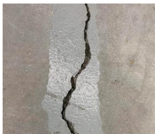
Figure 4. Large Crack.
