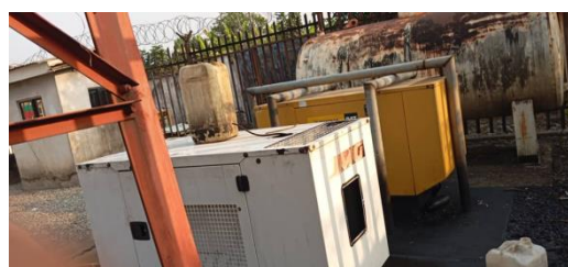
Figure 4. The two generating sets operating 24/7 hrs in the base station.
