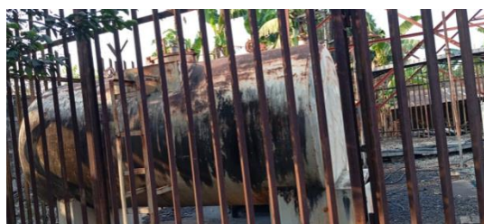
Figure 6. Diesel Storage Tank without Bundwall.
