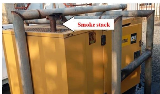
Figure 5. The location of the generators smoke stack.
