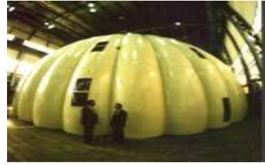
The wave-shaped surface: the glass-reinforced plastic umbrella shell GRP (OAO «Avangard»)
