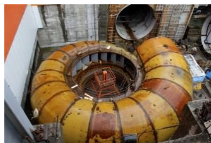
d) helical-shaped surface (spiral camera of hydraulic turbine of water-power station is a settling name but with geometrical point of view this is not correctly)
