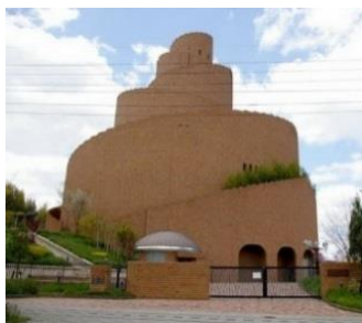
c) ruled spiral surface (water tower "Kizuminami", Kizu, Japan, 1999 [bugaga.ru/interesting])
