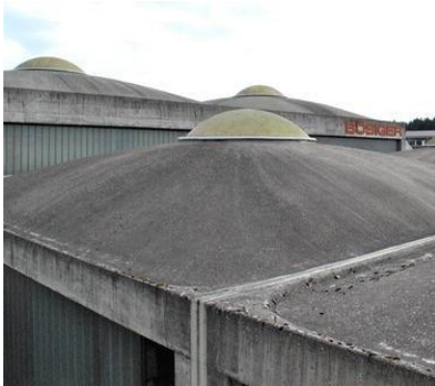
a) the funicular shell formed by the chain lines (Heinz Isler)
