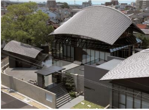
c) roofs from corrugated iron in the form of cylindroids (Ishibashi, Tokugawa & Associates, Токио, Japan)
