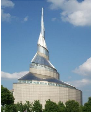
c) a torse surface with an cuspidal edge on a circular cone (spiral-shaped roof)
