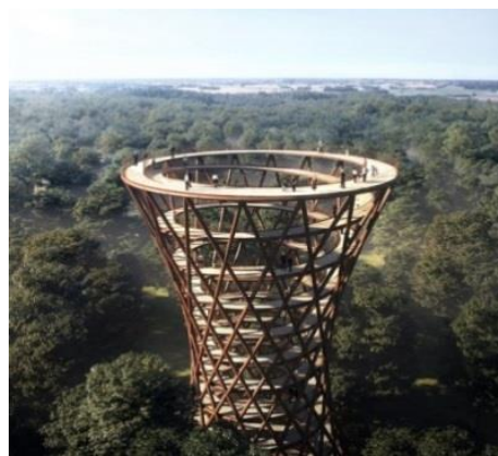
b) a project of footpath of the studio Glissfeldt Kloster, Denmark, with a director spirale on the one sheet hyperboloid of revolution
