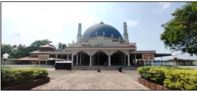
Figure 5. Pidie-Labui Grand Mosque, Source: documentation, 2024.
