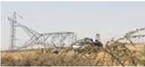
Figure 7. Vandalization of high voltage power line.
