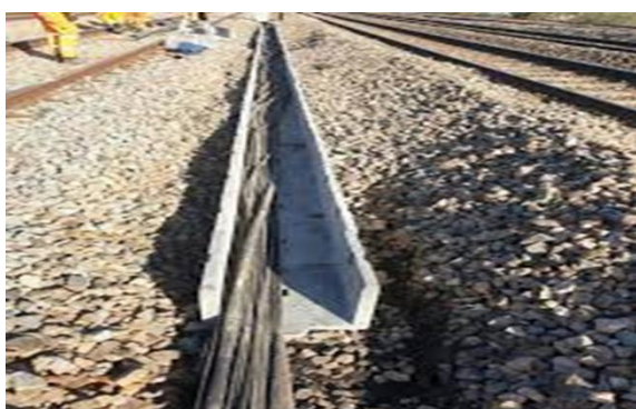
Figure 15. Telecommunication Corridor along Rail Tracks.
