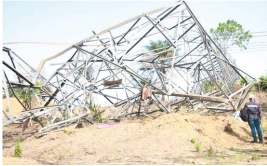
Figure 6. Vandalization of high voltage power line.
