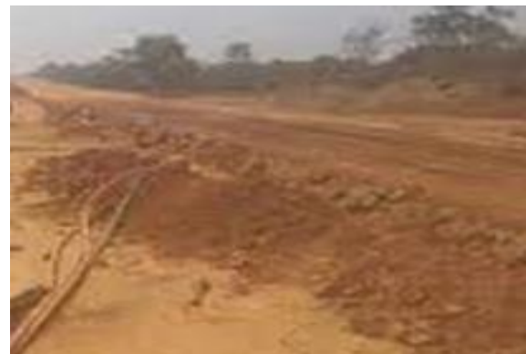
Figure 5. Vulnerable optic fibre cables during road construction.
