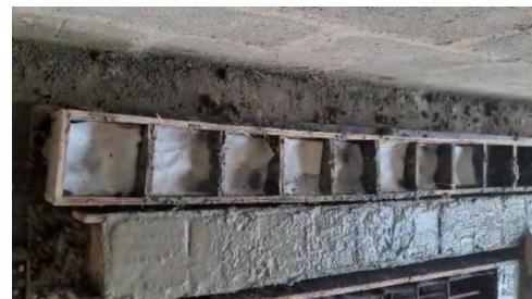
Figure 1. Image Showing Concrete Cubes with Geotextile at the Middle.
