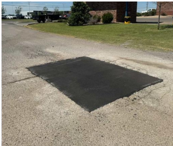
Figure 4. Patching and repairing a road pavement.
