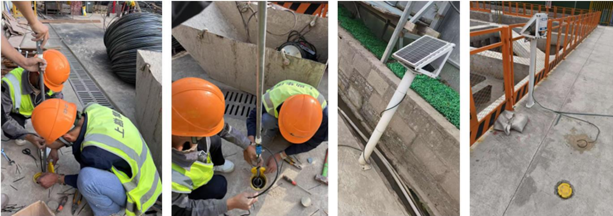
Figure 10. On-site installation diagram of automatic inclinometer equipment.
