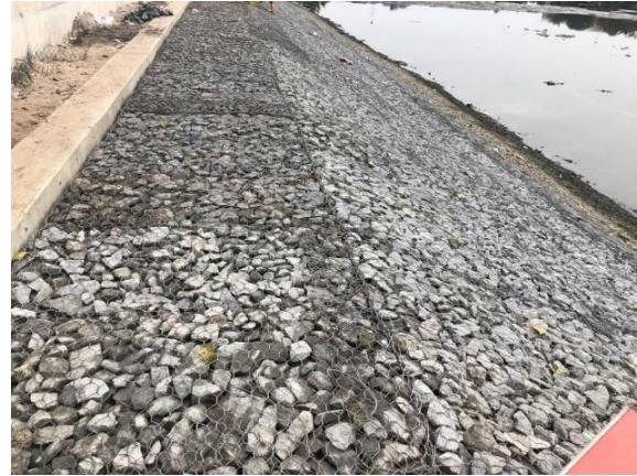
Figure 8. Fully constructed shoreline protection.
