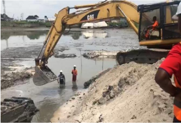
Figure 5. Placement of crushed stone footing.
