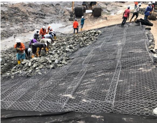
Figure 6. Filling of gabion gauges with crushed stones.
