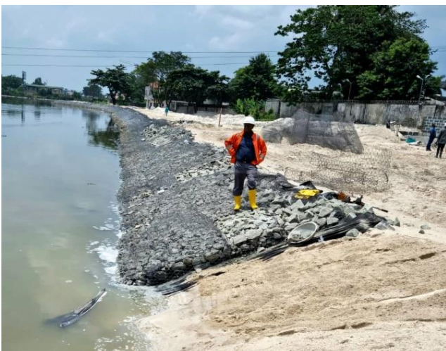
Figure 7. Partly constructed Gabion revetment.
