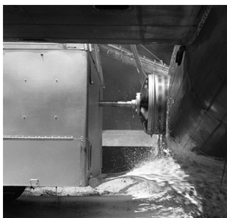
Figure 26. Testing of a special hole saw as part of the Monegeeta Monster programme (1948-1950 [14]).
