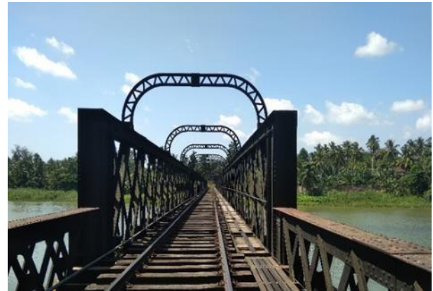
Figure 16. Katugastota Railway Bridge.
