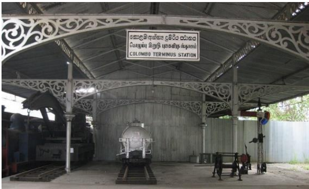
Figure 2. Cast iron brackets, Terminus Station.
