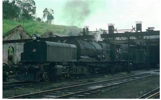
Figure 11. Old Running Shed, Nawalapitiya.
