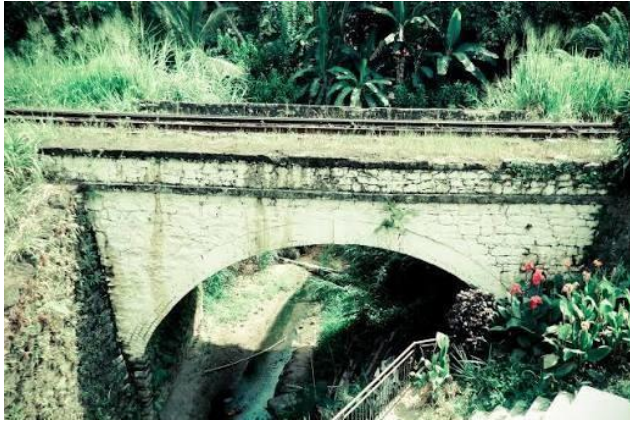
Figure 15. Nanu Oya Arch bridge.
