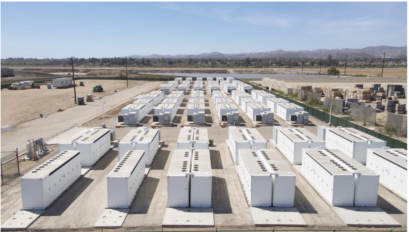
Figure 5. The Tesla Megapack battery storage-based Saticoy battery storage system, with a capacity of 100MW/400MWh, was launched last year.
