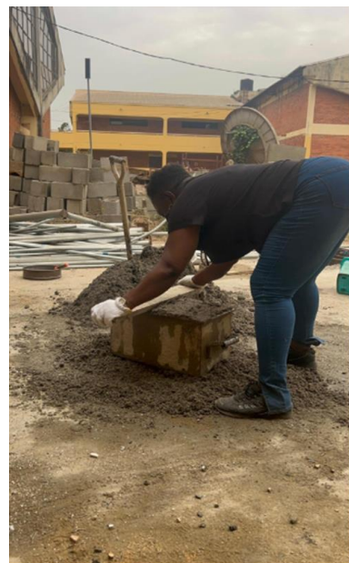
Figure 15. Casting of Blocks.
