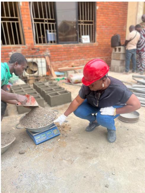
Figure 13. Batching Process.
