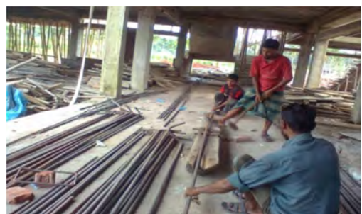
Figure 15. Construction workers doing risky work without taking any personal protective equipment.
