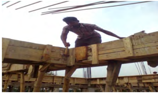
Figure 16. Working without safety net and helmet.
