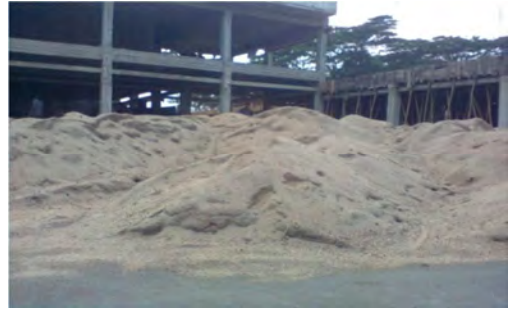
Figure 12. Uncovered sand deposit.
