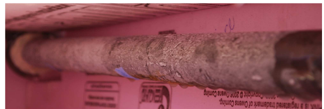
Figure 18. Evaporator pipe with condensation enclosed inside an insulated box.
